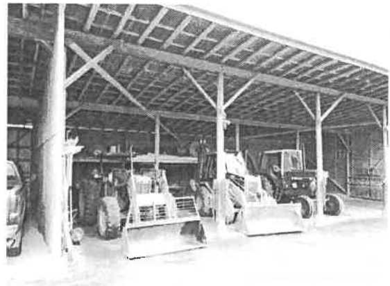
Client Provided Photos
