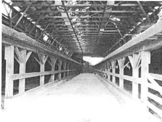
Client Provided Photos
